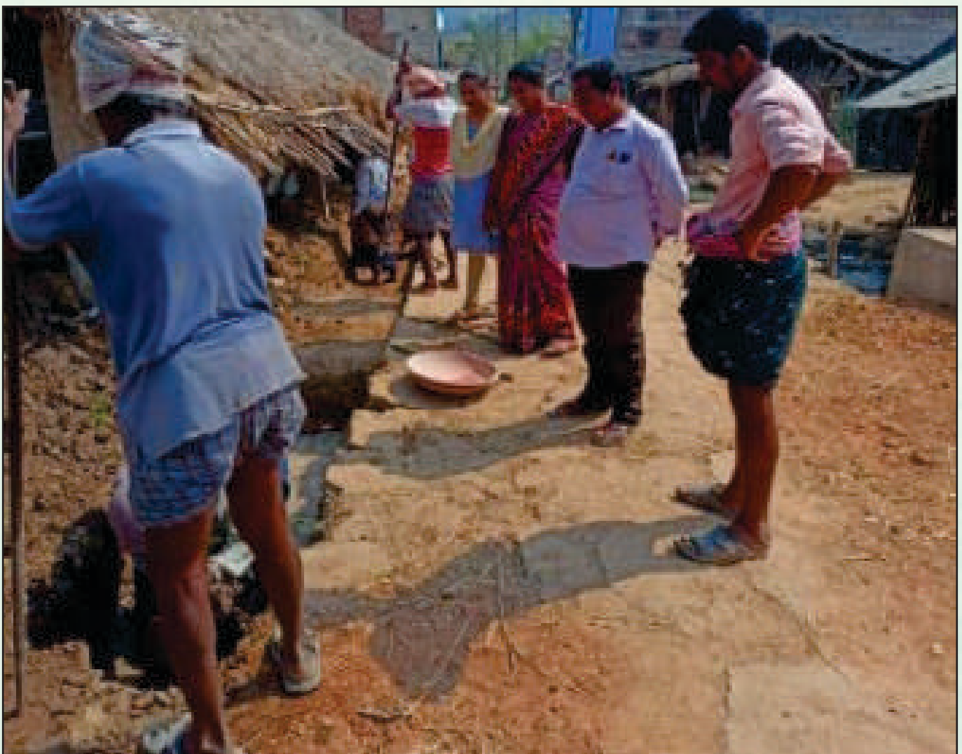
Drainage work Under Progress
