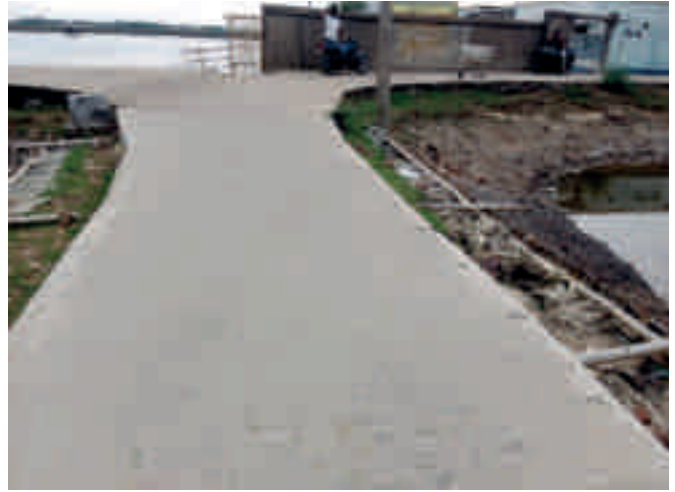
After CC Road constructed
